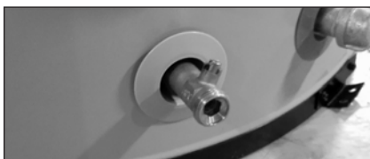
Figure 45 - Drain Valve.
