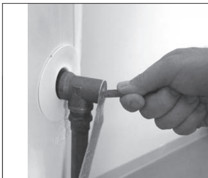
Figure 49 - T&P Relief Valve.
