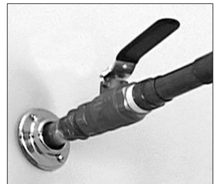
Figure 20 - Fully open the cold water supply valve (full-flow ball valve pictured above).
