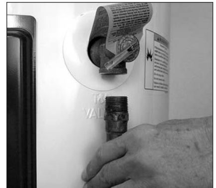
Figure 12 - Removing the T&P Relief Valve discharge pipe.
