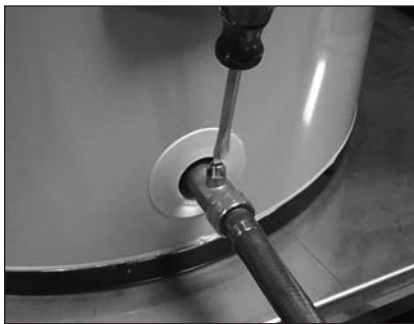
Figure 11 - Draining the old water heater.
