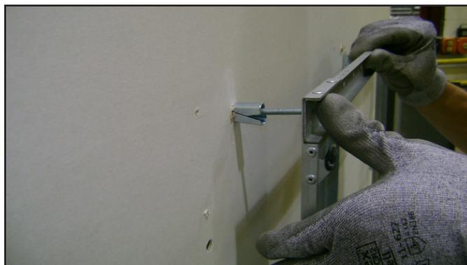
Figure 4.11 Installing Anchors in Hollow Wall
