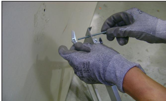
Figure 4.10 Toggle Bolt Installation through Mounting Bracket
